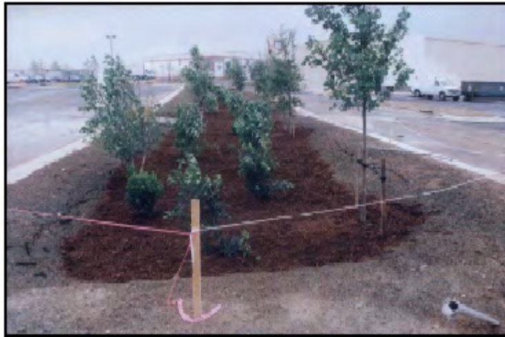
Newly Constructed Bioretention Area
