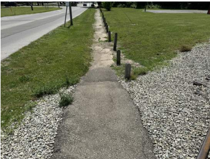
Non-accessible walkways at Industrial Park
