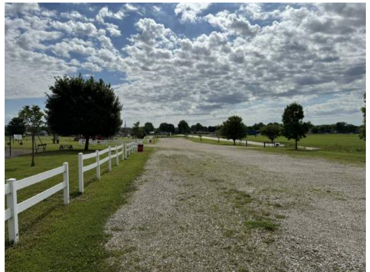
Gravel parking lot at Soccer Complex
