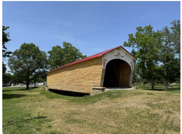
Covered bridge at Roberts Park
